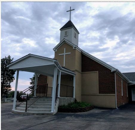
Sept/2018 Newly Renovated Entrance
