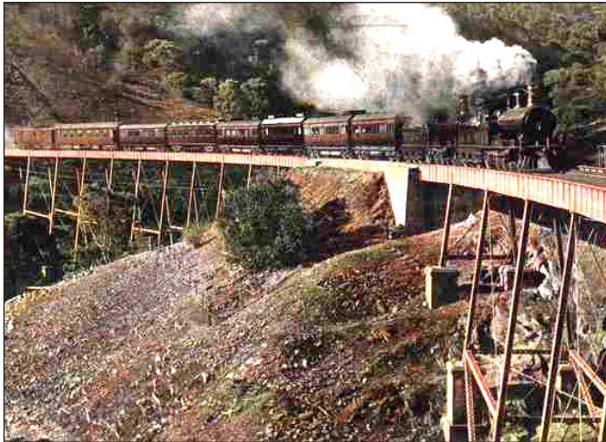
Sleeps Hill Viaduct Eden Hills 1907, Courtesy CV&DNT
