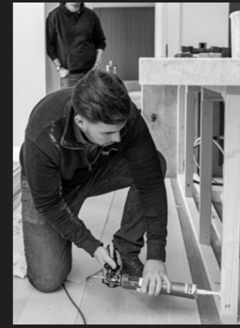
Building support structure
