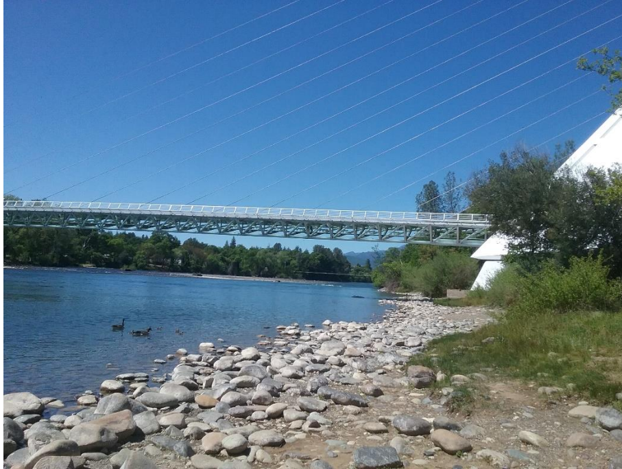
The Sundial Bridge in Redding, CA is similar to a wildlife corridor, but it's for people. The architect Santiago Calatrava designed the bridge so that no piers would enter the Sacramento River, preserving a corridor rather than restoring it.
