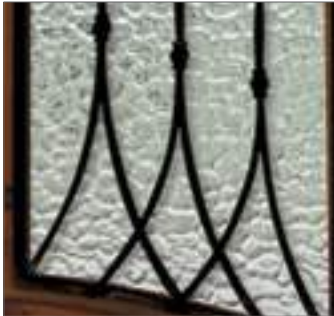
Detail photo of Warwick wrought iron grille,
