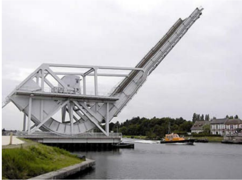
Scherzer Rolling Lift design partially opened. Notice that span has further to 'roll' to open to a greater degree.
