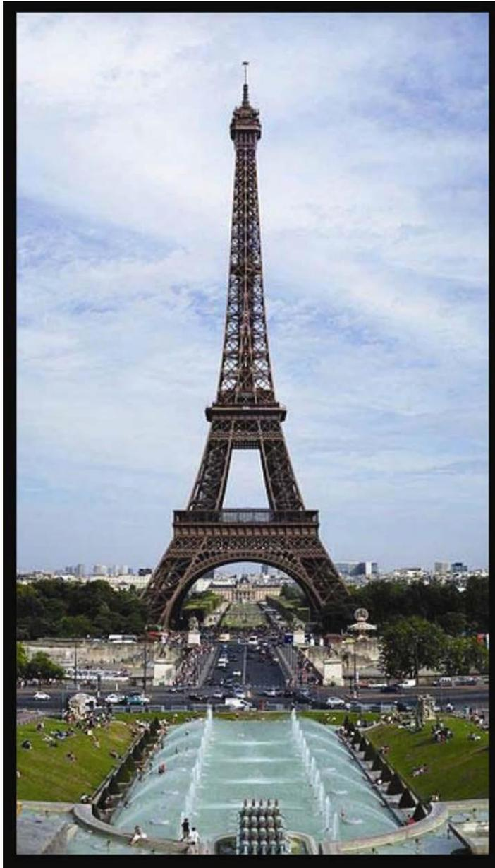
tall, stiff tower with an extremely high margin of safety against wind loading conditions. It was this feature that effectively made the tower a tour-de-force of engineering design for the age.
