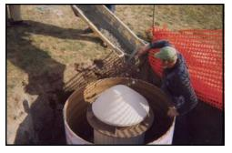
Once in place, the entire void between the old deteriorated wall and the plastic covered forms are filled with highstrength ready-mix concrete.
