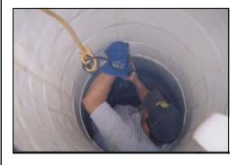
After the concrete has set, the formwork is disassembled. The joints then receive a heat-fused welding strip to completely seal the new concrete from future corrosion. Then the liner is spark tested to ensure there are no defects or pinholes.
