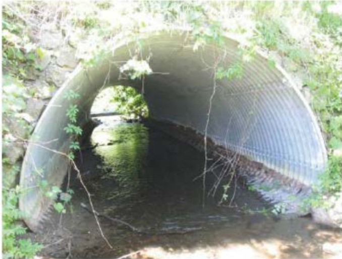
Top right, bottom right: After pipe rehab
