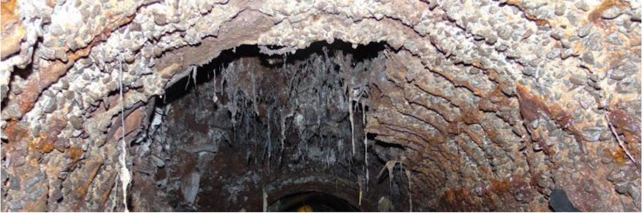
*Top half of interceptor, completely rotted out and held in place by root masses*
