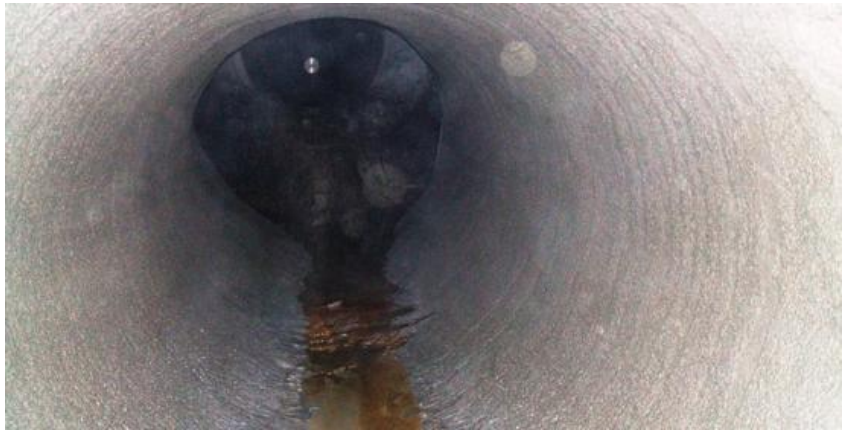
The rehabbed pipe is waterproof, smooth and relatively thin, so flows are not restricted.
