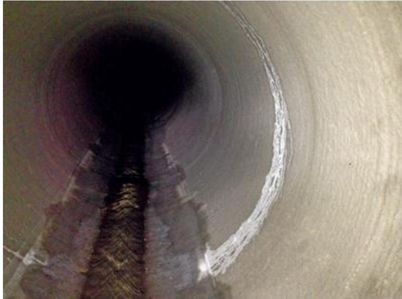
*As of July 2015, AWC has completed work on four of the seven highway culverts using the centrifugally cast concrete pipe (CCCP).*
