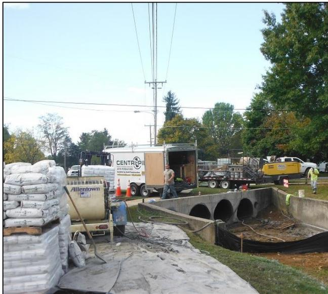
**The culverts that required repair ran under one of the main thoroughfares in the town, making it less than ideal to close the street completely during the work.**
