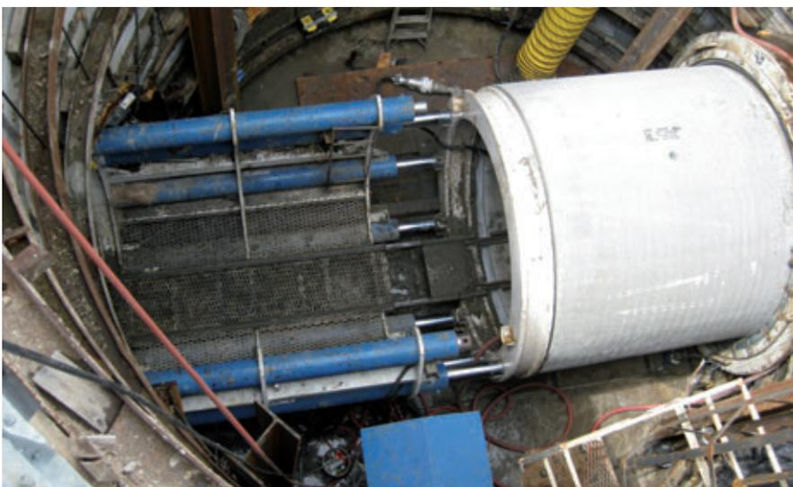
*The bid-winning contractor, SAK Construction LLC, decided to use 96-inch pipe, rather than the specified 90-inch, in order to use a tunnel boring machine (TBM).*
