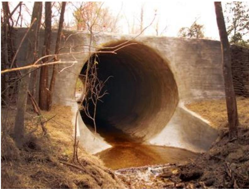
In March 2010, an unusually configured culvert passing under Florida State Route 16 was rehabilitated with a solution called CentriPipe, utilizing PL-8000 fine aggregate composite concrete developed by AP/M Permaform. Florida Department of Transportation (FDOT) has been monitoring the project
