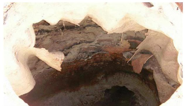
Nearby manhole without Con<sup>MIC</sup>Shield<sup>®</sup>. Epoxy has delaminated.
