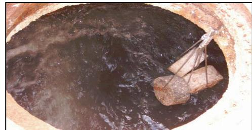
The manhole shown below is only 15 feet away from Manhole #40. The epoxy coating peeled off as shown below.
