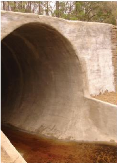
The pipe after project completion
