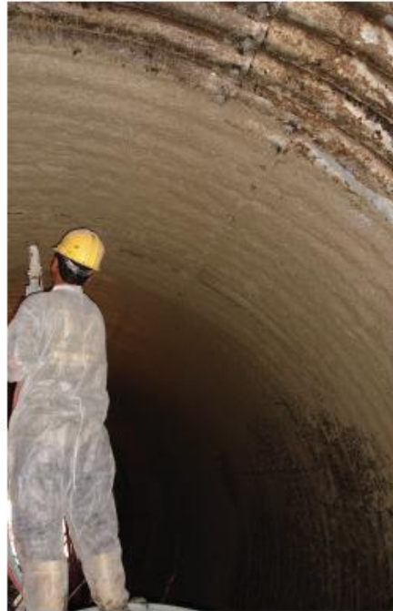
Transfield Services North America
