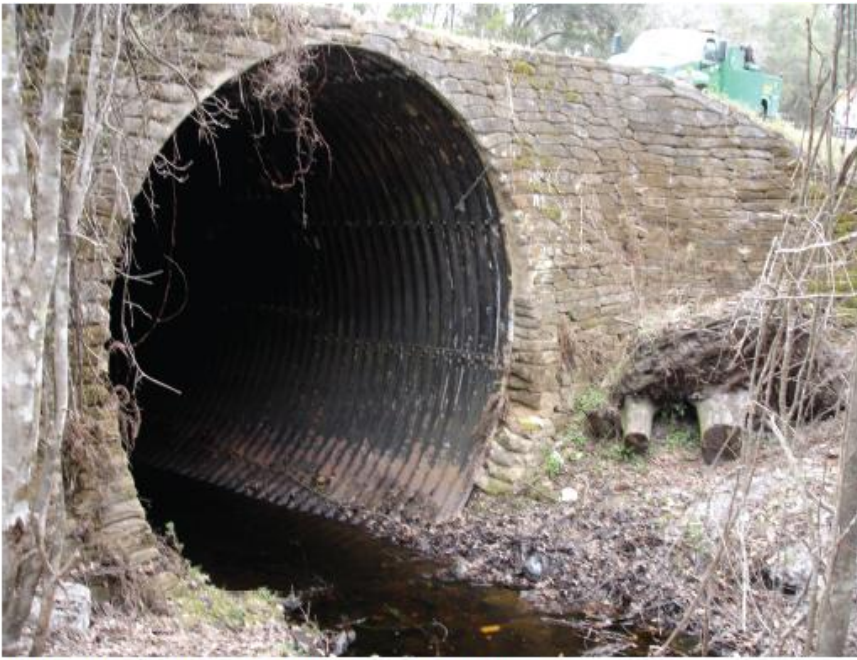
The Clay County culvert pipe before the project began
