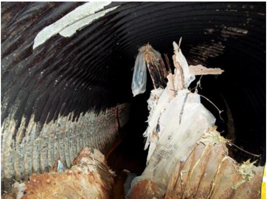
The 66-inch culvert collapsed even further between quote and award. There were completely corroded inverts and sidewalls curling up into the interior.
