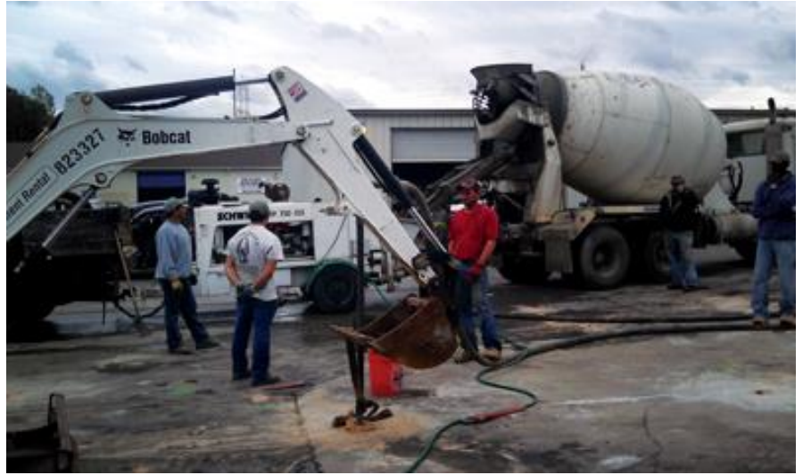
To prevent soil instability, the team stabilized the surrounding soil with cementitious grout.
