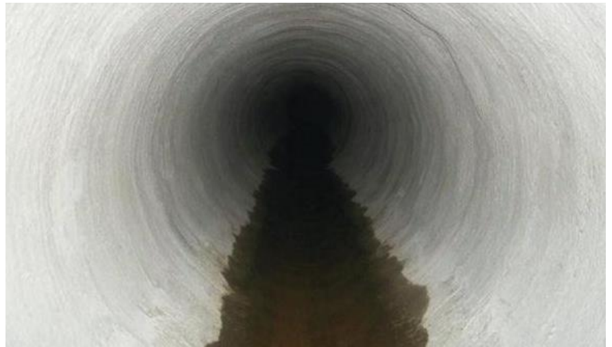
The corrugated metal was lined with four-part steel rings, each 18 inches wide, which were then sprayed with high-strength cementitious grout for a smooth, watertight finish.
