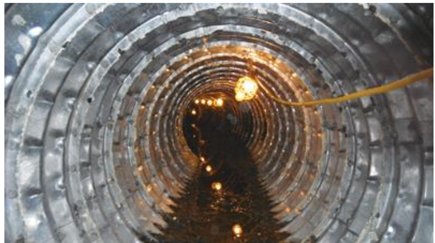
In phase one, 54-in. tunnel liner plates were used to structurally stabilize the culvert.
