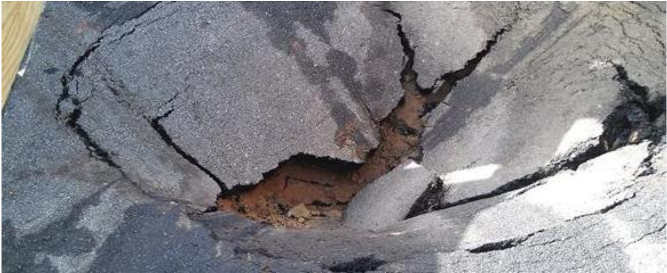
Parking lot sinkhole above collapsing CMP in Clayton County, GA
