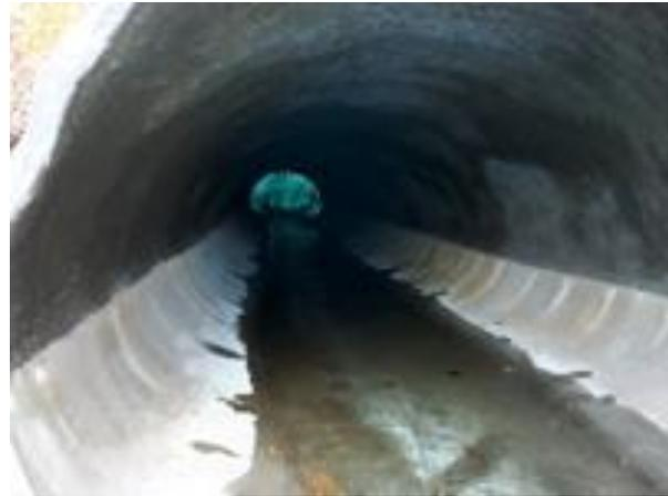
*A completely rehabilitated arched metal culvert; the upper arch was spraycasted with cementitious grout.*
