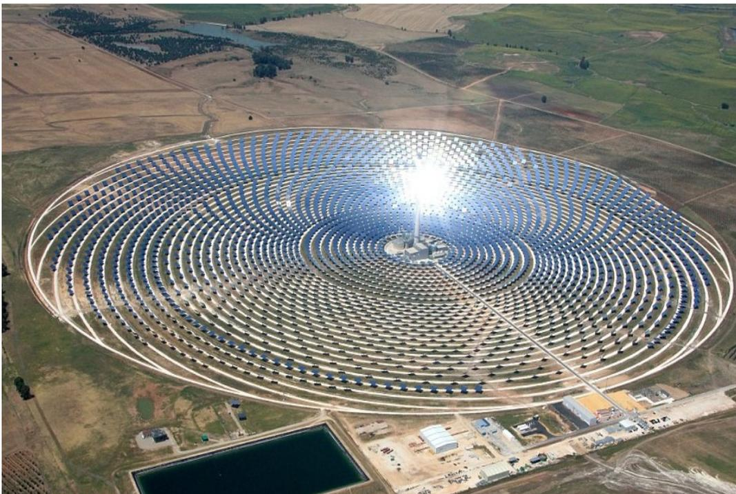
A Concentrated Solar Power Plant with an array of mirror-lenses that heats water on a central column.
