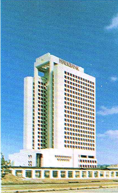
Construction of high rise building 67 000 sq.m., floor area, 30 floors.
