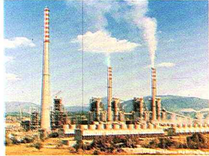
Turnkey construction of 6x165 MW Soma-B Thermal Power Plant
