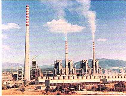
Turnkey construction of 6x165 MW Soma-B Thermal Power Plant
