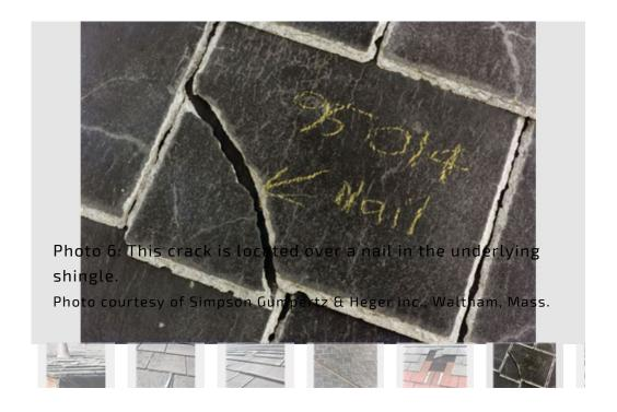
Before the 1980s, most artificial roofing slate was made from asbestos-cement, a material that had a long track record of successful performance. When the use of asbestos became forbidden, manufacturers rushed to replace asbestos-containing products with cement-based products reinforced with nonasbestos materials.
