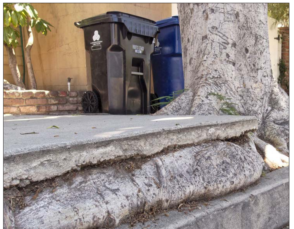
A tree root causes sidewalk damage.
