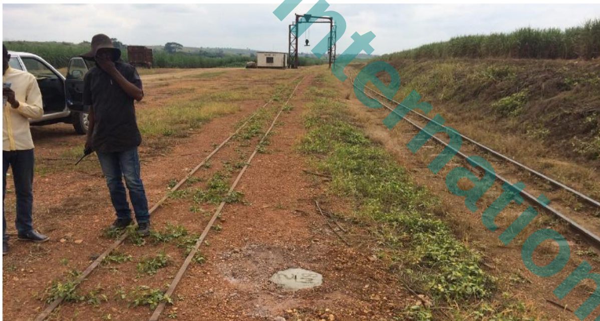
Image 7: Installing a Ground Control Point and measuring the point with the GPS Rover.
