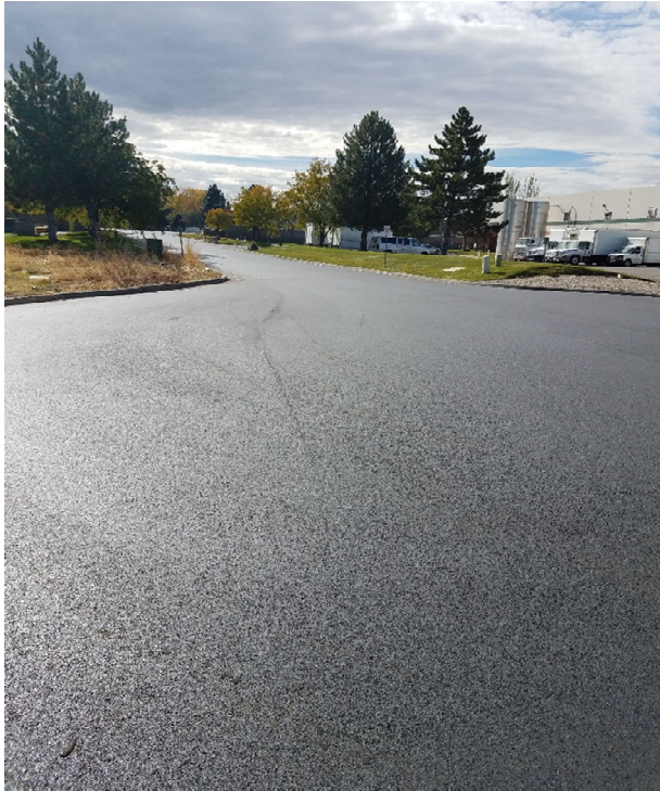
Final 2" Overlay (2940 West Culd-de-sac)
