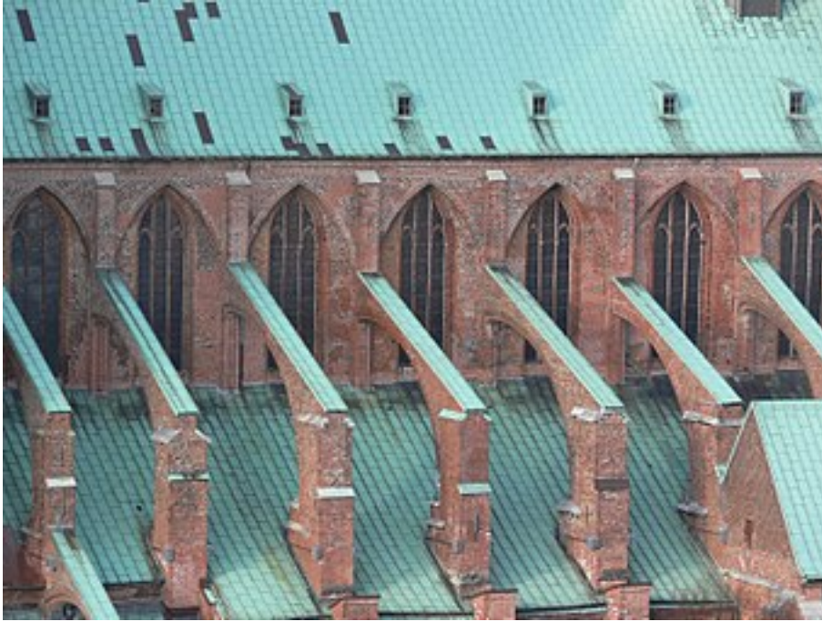
Flying buttresses support the main vault of St. Mary's Church, in Lübeck, Germany.
