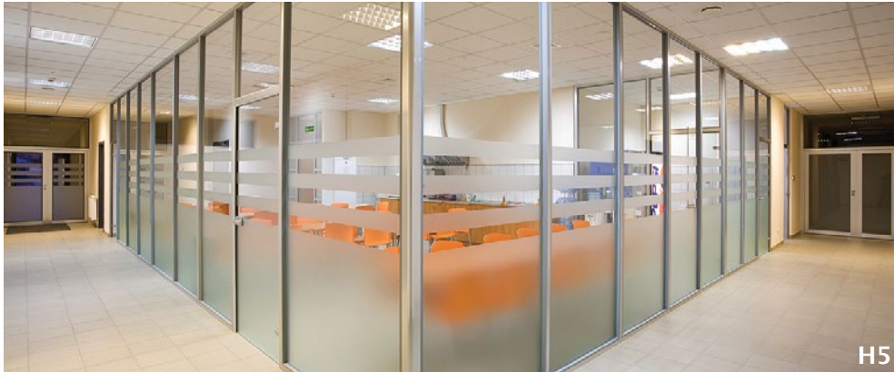
Frame: Full-height glass panels encased in vertical aluminum extrusions
