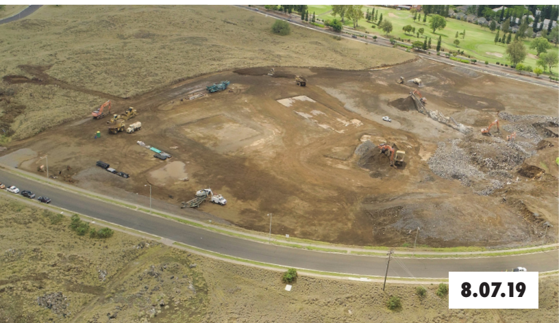
2 months of mass grading by the construction team, defining the boundary of Waikoloa Plaza.
