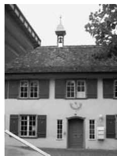
Steigstrasse 26, Altes Casino
