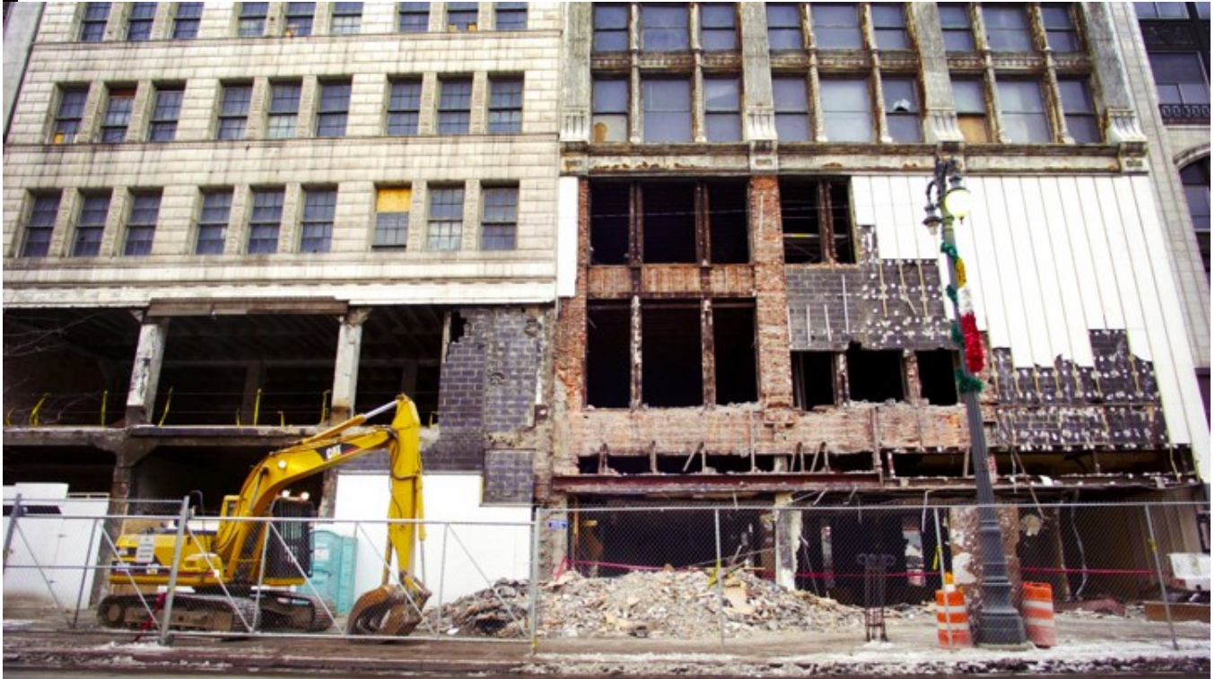
Construction in downtown Detroit (PAUL SANCYA / AP)
