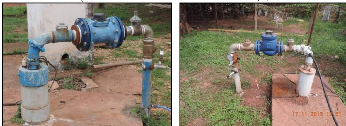
Figura 3. Barrilete do PT-01 (A) e PT-05 (B) (A) (B)
